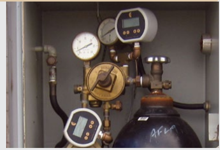
Substation Transformer Nitrogen Blanketing
